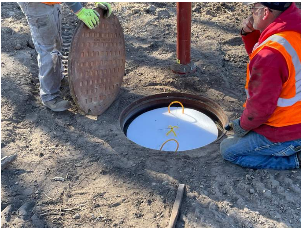
Photo #2: Insulation caps installed in the AV/AR manholes - Mar 18, 2024, 10:22 AM
