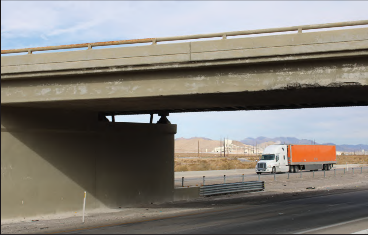
VIEW OF ROUND NOSED PIER
