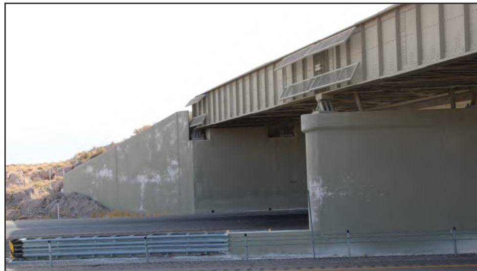
VIEW OF ROUND NOSED PIER
