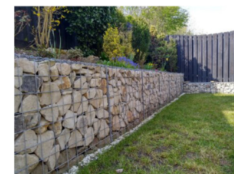
ROCK-FILLED GABION BASKETS
