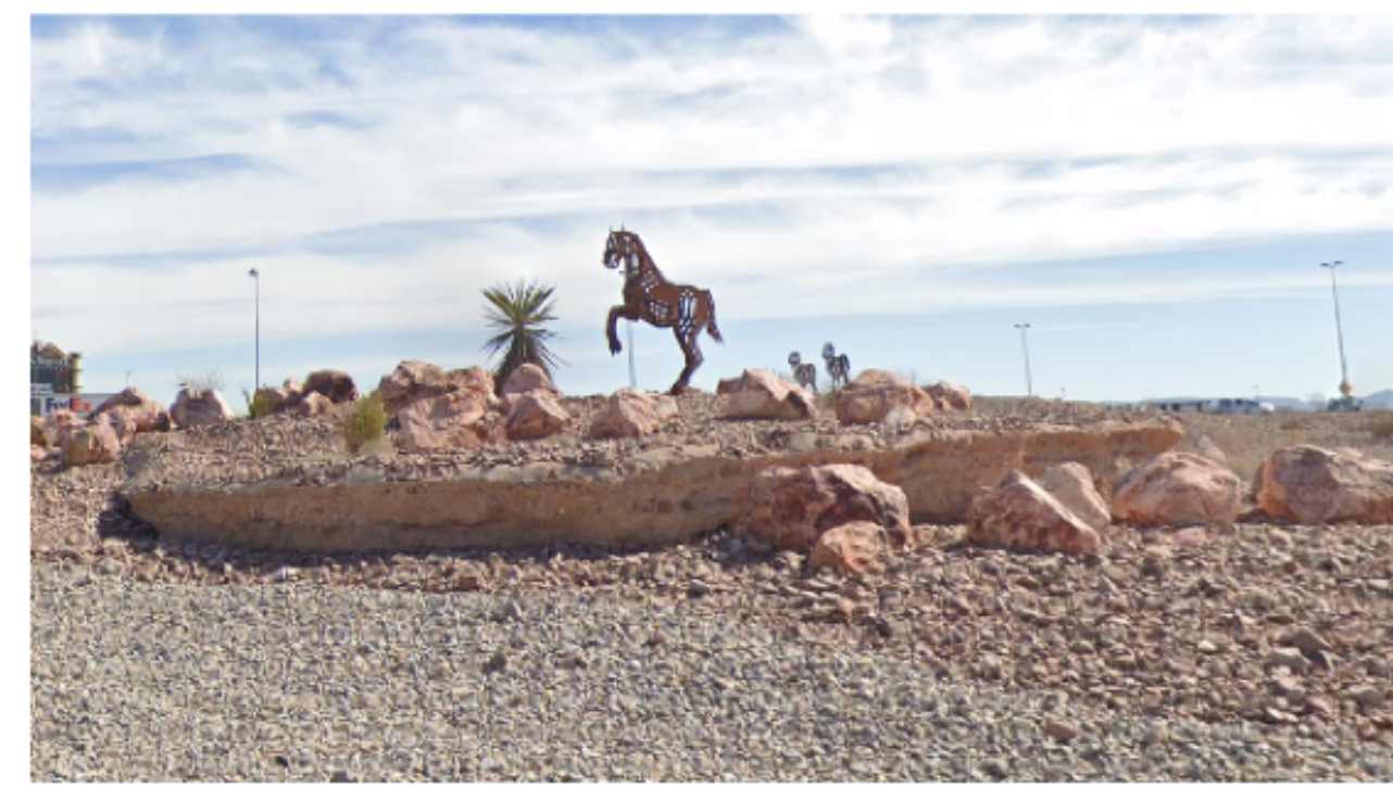
FAUX RAMMED EARTH ACCENT WALLS
