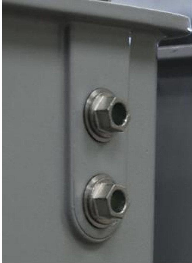
Old Fiber Entry Ports
