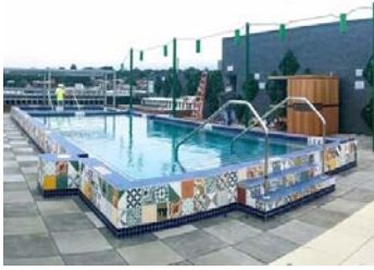
Concrete Renovation City Club Apartments Kansas City, MO
