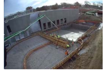
Swimming Pool Merriam Community Center Merriam, KS
