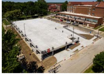
Parking Garage Donnelly College Parking Garage Kansas City, KS
