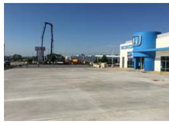
Conversion to Concrete Dale Willey Honda Parking Lot Lawrence, KS
