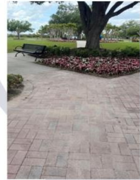
The pavers have been fixed
