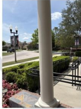
The pillar has been fixed and freshly painted
