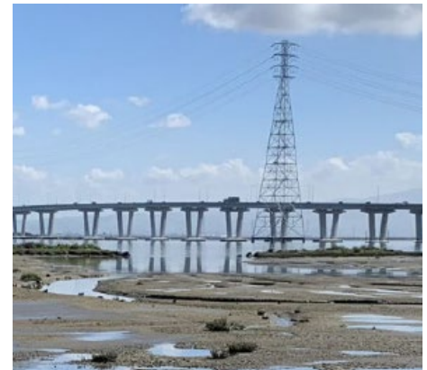
Western span of Dumbarton Bridge on a sunny day.
