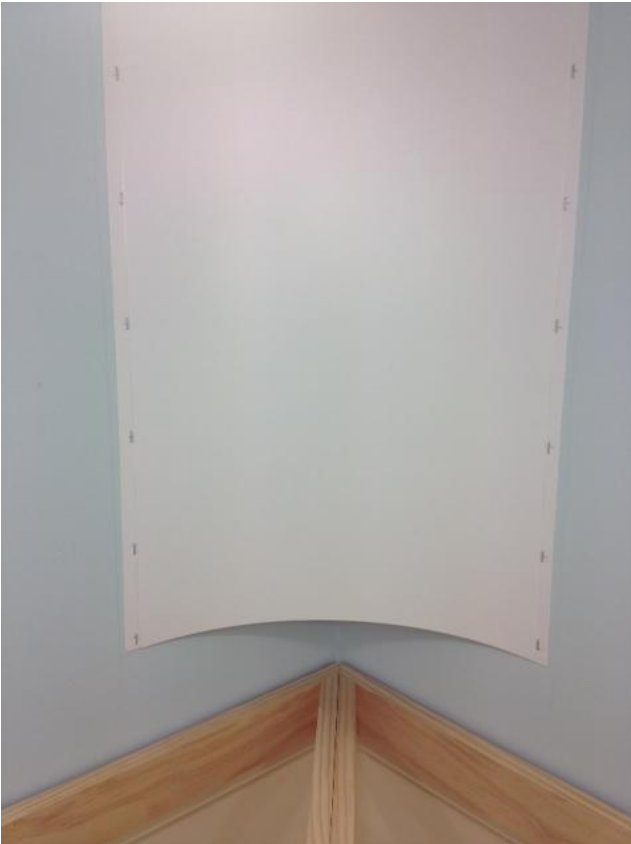
▼ .040 styrene forms the coved corner
