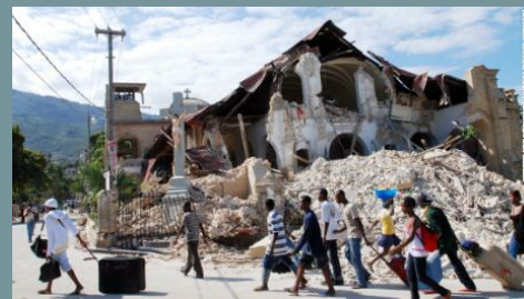
Aftermath of earthquake in Haiti.
