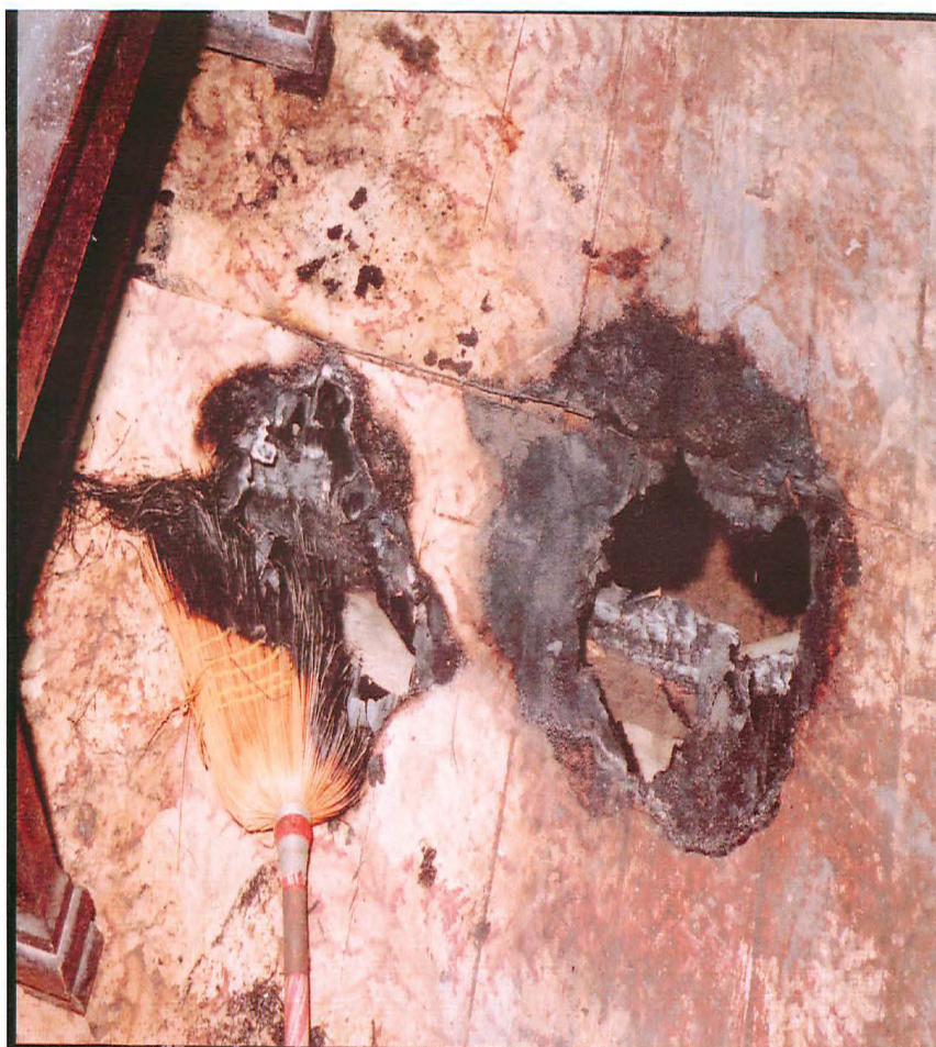
Figure 1. Two holes burned through the living room floor. A fire investigator opined that the fire burned in a smoldering state for 4 to 6 hours, thus challenging the veracity of the Defendant's alibi.
