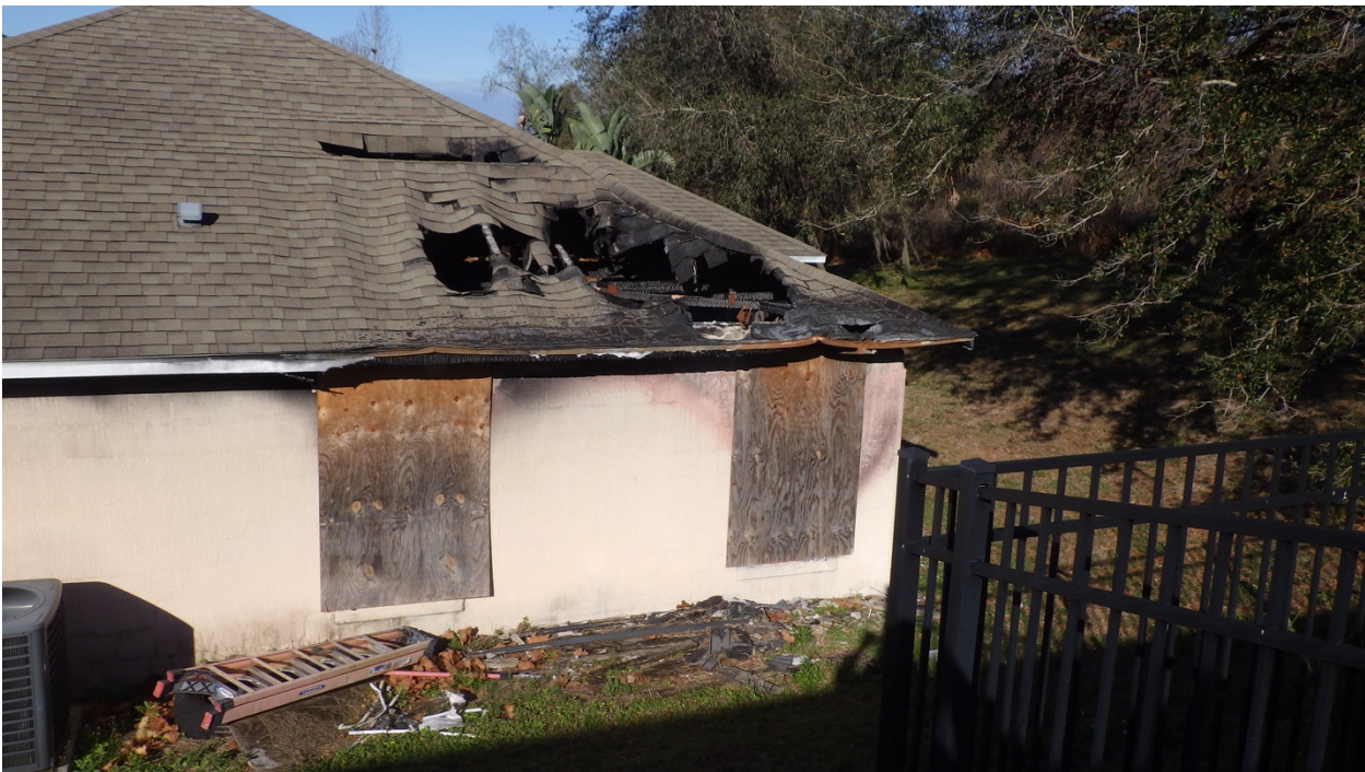
Figure 2. Burned roof above the room of origin.
