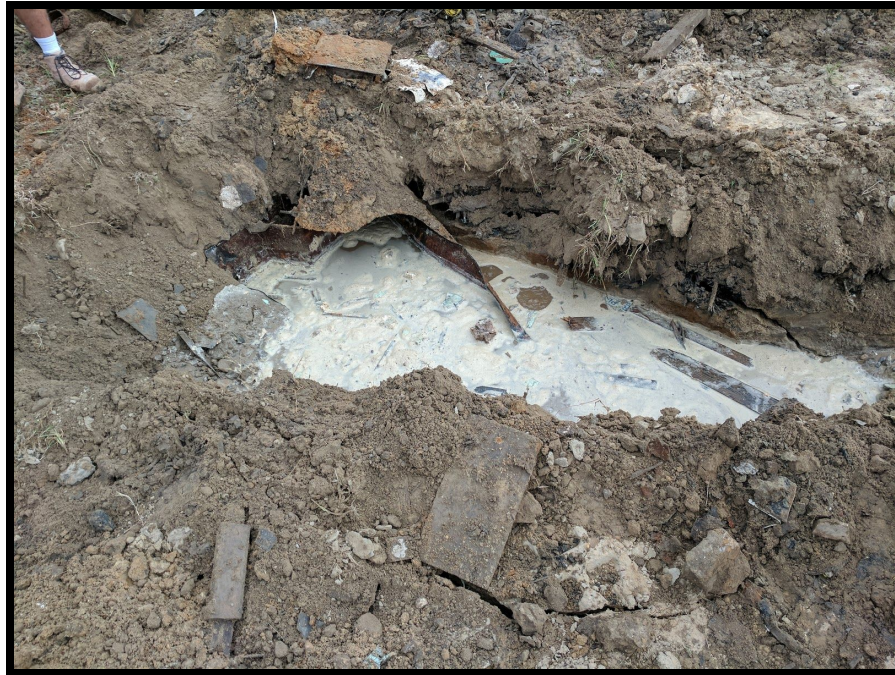
Old Septic Tank Below Grade
