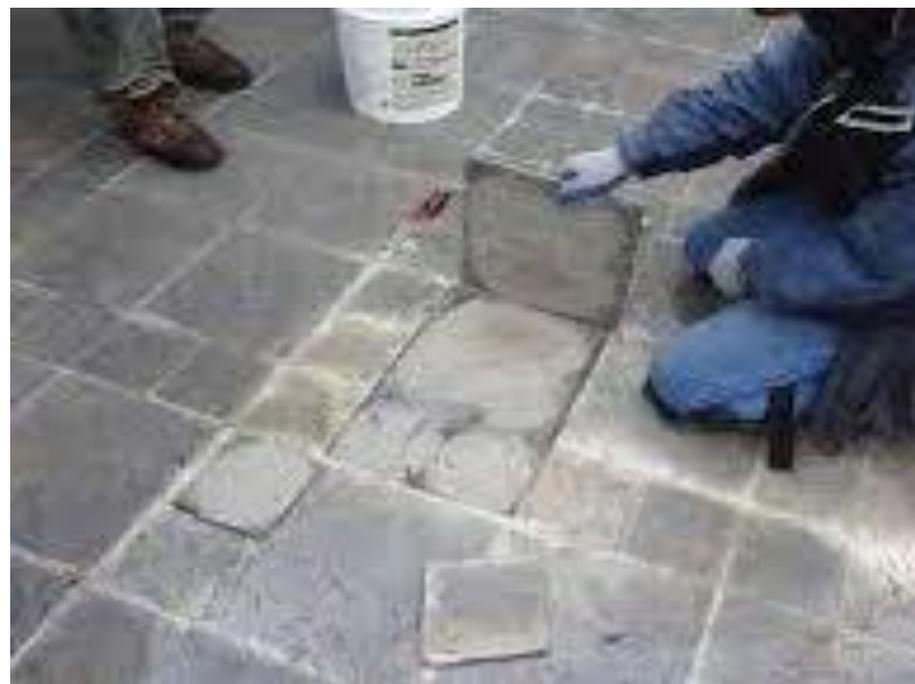
In colder climates, exposure to moisture can lead to problems associated to freeze/thaw issues. In warm climates, over time, moisture eventually “eats away” at the binding agents of mortars turning the setting beds to sand.
