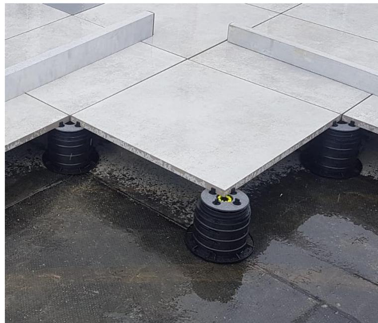
No. Applying pavers made of concrete (figure on left) on to pedestals has been around for a while. These applications are very common on the roofs of hotels, apartment complexes, around pool decks and so forth. What is new is that the ceramic tile industry has developed porcelain pavers as an alternative to concrete pavers which have many more benefits such as being thinner, lighter and non-absorptive.
