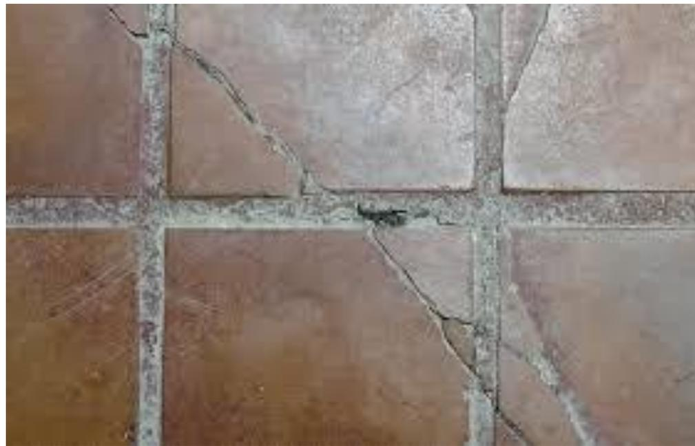
There are a multitude of benefits associated to exterior raised floors. First, tiles placed on pedestals are not bonded, they are loose laid. As such, as opposed to “bonded” tile, there is no rigid attachment between tile and structure, therefore, structural forces cannot “crack” the tile.
