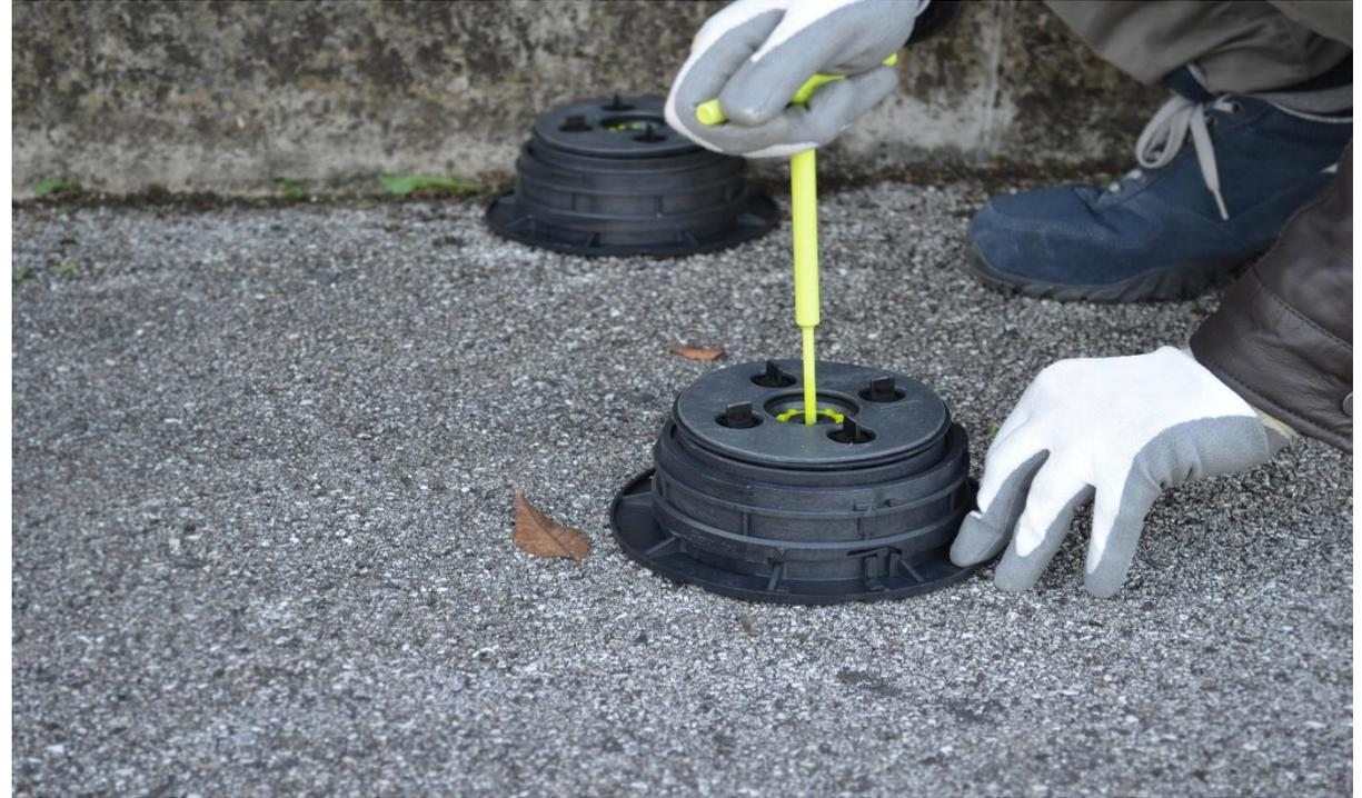
As opposed to adhering tile directly to a substrate, tiles are simply loosely placed on top of a series of pedestals generally situated at each corner of the tile. This is possible with the advent of 20 cm (3/4") porcelain paver tile, which can accept this type of weight and overall load.
