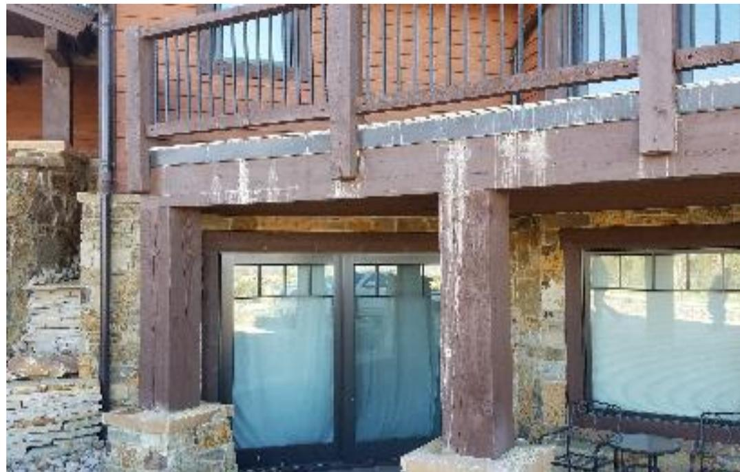
Other issues associated to “bonded” exterior tile assemblies? Efflorescence, which is the gradual leeching out of soluble salts (calcium) from setting beds on to the tile surface (picture on left) or adjacent building elements (picture on right).
