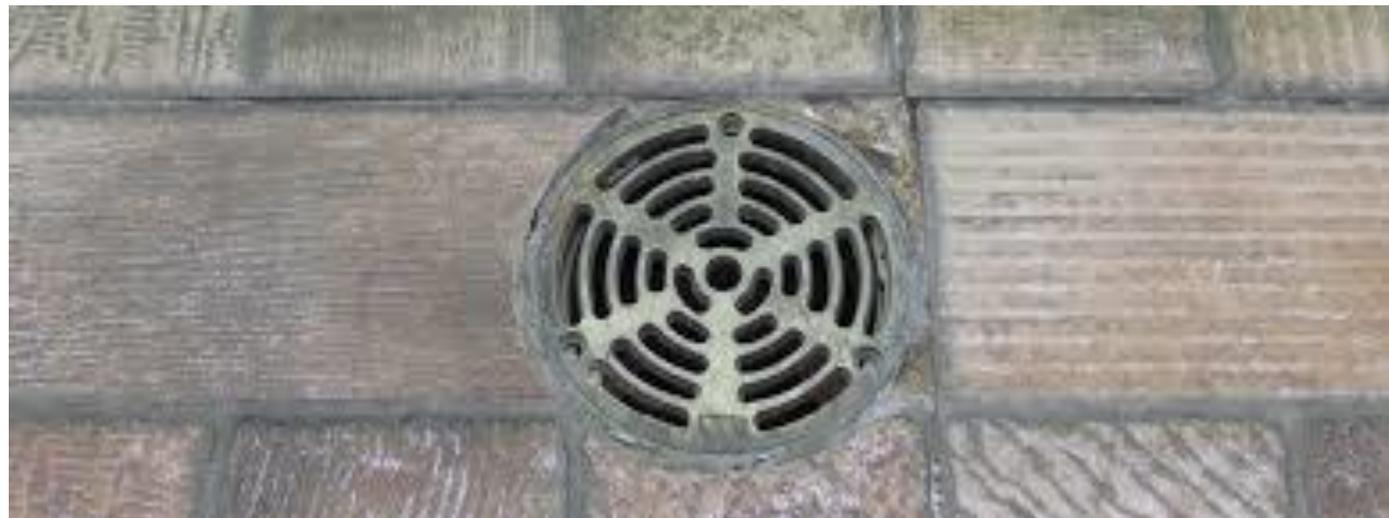
Since water drainage occurs under the tile layer, raised tile on pedestal installations are flat and continuous without grout joints, movement joints or visible drains. Traditional exterior “bonded” tile assemblies require a sloped surface, drains, grout joints and movement joints.
