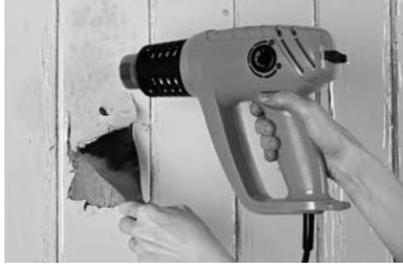
There is no way to eliminate dust, but some renovation methods make less dust than others. Contractors may choose to use various methods to minimize dust generation, including using water to mist areas before sanding or scraping; scoring paint before separating components; and prying and pulling apart components instead of breaking them.
