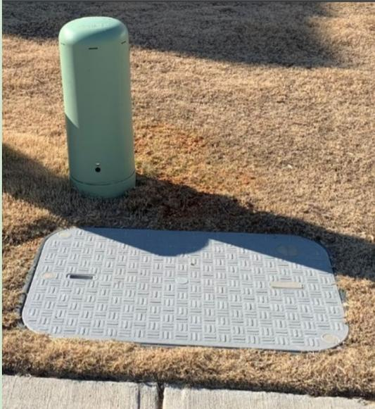
Crews contracted by Decisive Communications (main sub for Spectrum) will arrive about one week after the utilities are marked and begin the process of boring and digging the underground line, installing the “vaults” at the major connections and installing “pedestals” every two homes for the service connections to homes. Crews will work to restore and clean up the impacted areas behind the installations.
