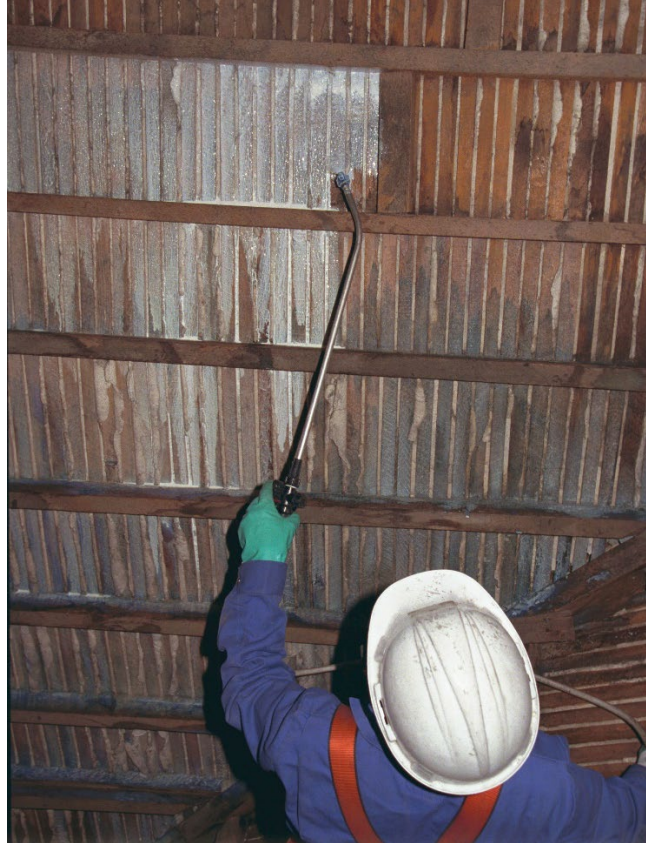
Figure 14: Initial application of consolidation agent. (Notre Dame Cathedral, Ottawa)
