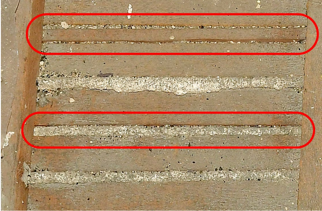
Figure 2: Non-viable keys. In the uppermost red circle, the lath spacing is too narrow for a functioning key. In the lower red circle, there was not enough squeeze-through to form a functioning lug.
