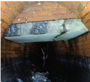
Deteriorated brick sewer before QLS.
