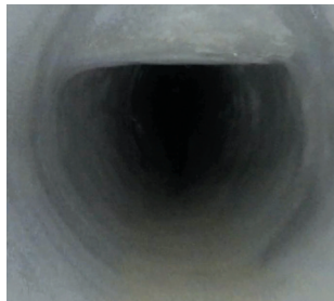
Brick sewer structurally restored utilizing QLS.
