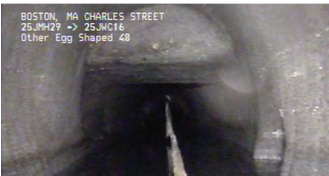
Same brick sewer one year after QLS installation.
