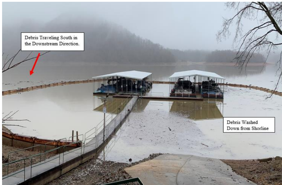
Figure 5: Verification of Debris Traveling in Direction of Wind and Water Vectors
