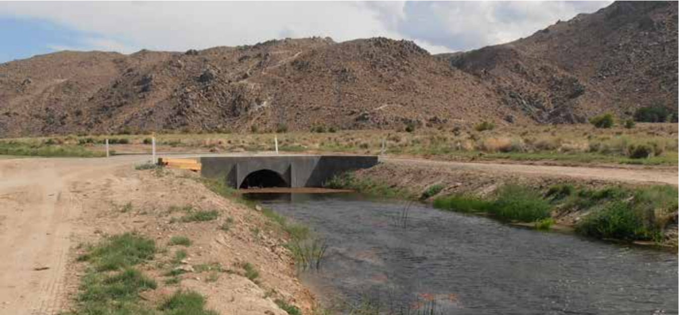
New Check Wall and Road Crossing in the Big Pine Canal (July 2014).
