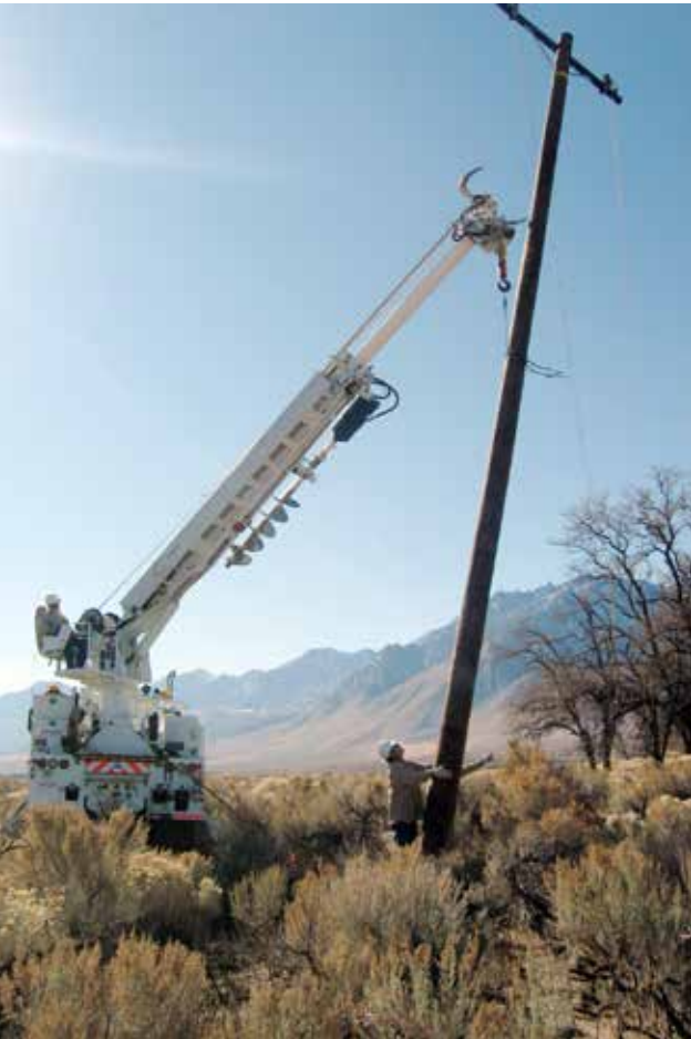
Hines Spring Well 355 Project (November 2011) LADWP Erecting Powerline to Power Well 355
