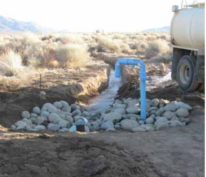
Pipe Outfall (convergence of both pipelines) Within Exclosure During Implementation, December 2011
