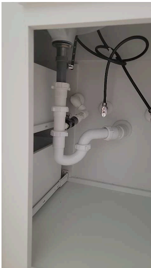
CLIENT INFORMATION: This is a picture of the AC primary condensate drain line that discharges into the plumbing drain line under the sink. This was noted in the front downstairs bathroom in the secondary bedroom. CLIENT INFORMATION: This is a picture of the AC primary condensate drain line that discharges into the plumbing drain line under the sink. This was noted under the left sink in the master bathroom.
