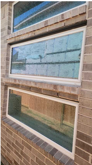
These window lintels were noted behind the master bathtub.
