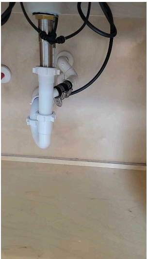
CLIENT INFORMATION: This is a picture of the AC primary condensate drain line that discharges into the plumbing drain line under the sink. This was noted in the front downstairs bathroom in the secondary bedroom. CLIENT INFORMATION: This is a picture of the AC primary condensate drain line that discharges into the plumbing drain line under the sink. This was noted under the left sink in the master bathroom.
