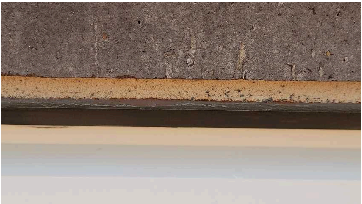
These window lintels were noted behind the master bathtub.
