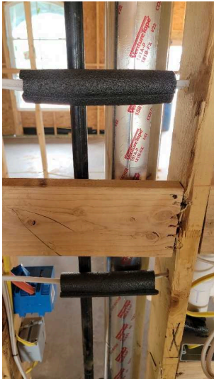
I observed a missing nail plate at the blocking for the cabinetry at the time of the inspection. A nail protection plate helps prevent nails from piercing pipes and electrical lines after the drywall is installed and the finish trim is being applied. Nail protection plates are typically installed over utilities that pass through framing members. The blocking used for cabinetry fasteners tend to be longer than the standard 1 1/4 inch drywall screws which has the potential to cause damage behind it. This was noted in the kitchen opposite the laundry room. I observed missing fire blocking at the time of the inspection This was noted in the front hallway to the left when you walk in the front door.
