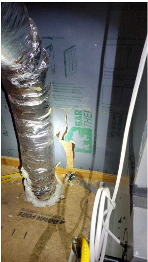
This was noted in the attic space.
