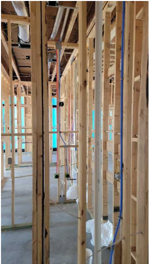
I observed a missing nail plate at the blocking for the cabinetry at the time of the inspection. A nail protection plate helps prevent nails from piercing pipes and electrical lines after the drywall is installed and the finish trim is being applied. Nail protection plates are typically installed over utilities that pass through framing members. The blocking used for cabinetry fasteners tend to be longer than the standard 1 1/4 inch drywall screws which has the potential to cause damage behind it. This was noted in the kitchen opposite the laundry room. I observed missing fire blocking at the time of the inspection This was noted in the front hallway to the left when you walk in the front door.
