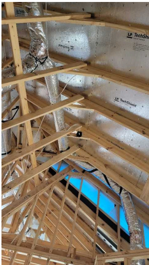
I observed the purlin was not flush with the rafter at the time of the inspection. A purlin is a horizontal structural member in a roof that supports a rafter. This was noted at multiple purlins in the back right corner when walking in through the front door.
