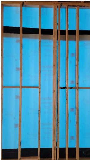
I observed missing fire blocking at the time of the inspection. This was noted in the interior wall of the garage. This was noted in the garage area on the exterior wall near the electrical panel.
