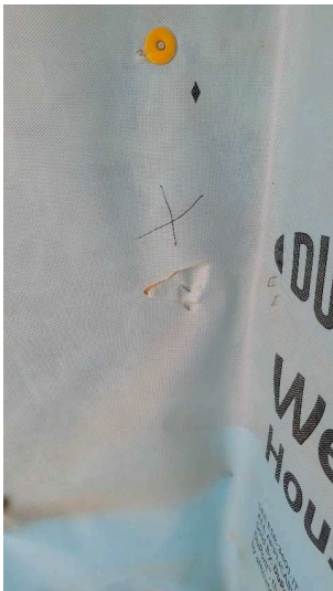
This was noted next to the window in the front porch area.
