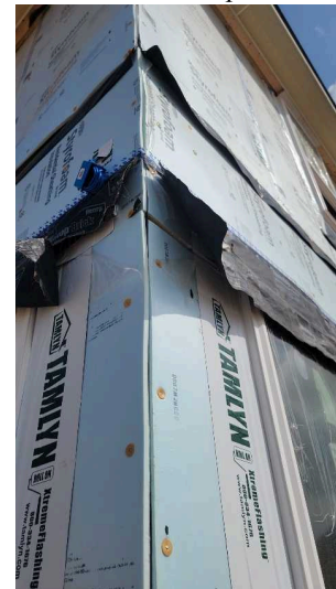
I observed a gap in the exterior structural sheathing I recommend it is sealed appropriately. This was noted on the left side of the home when facing the property from the street.
