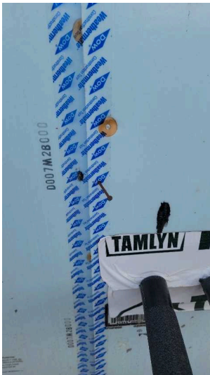
I observed a gap in the exterior structural sheathing I recommend it is sealed appropriately. This was noted on the left side of the home when facing the property from the street.
