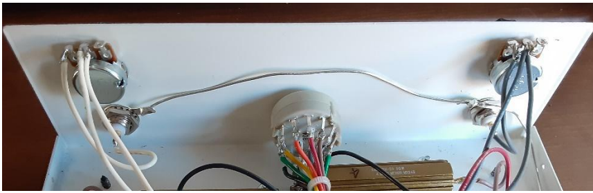
Figure 5 - Front panel wiring in place
