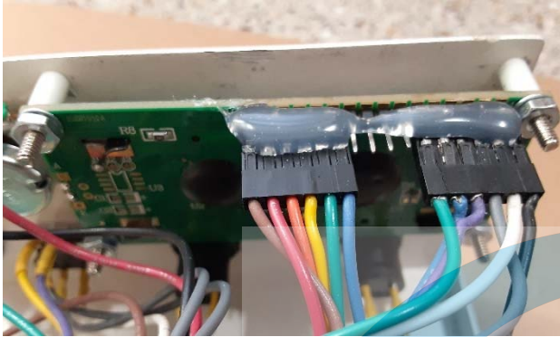
Figure 15 - Hot-glued wiring connectors
