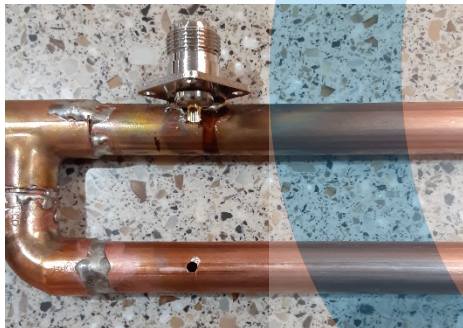
Figure 13 - Hole for wire drilled
