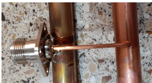
Figure 14 - 10AWG wire in place
