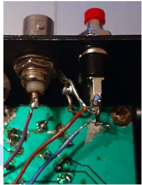
Figure 5 - Pushbutton switches as repaired
