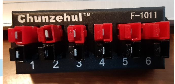
Figure 7 - Repaired distribution block
