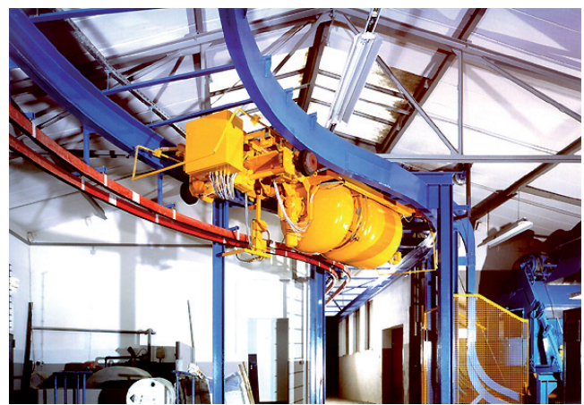
Feed and control of a concrete skipper
