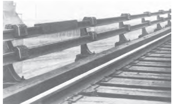
Typical Double Rail Installation
