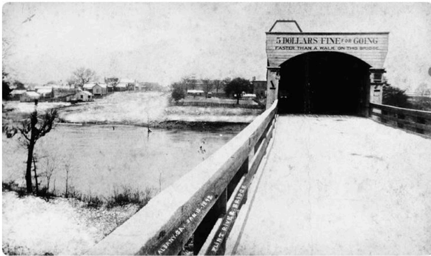
Flint River Bridge
