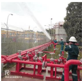
PERTAMINA EP CIREBON, 2019 FAIRBANKS NIJHUIS; 750GPM @150PSI, 5 UNIT,
