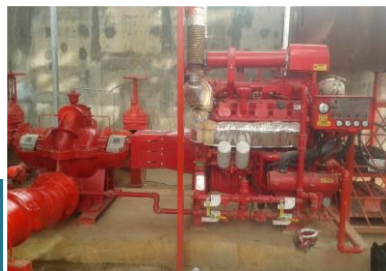
OKI - PALEMBANG, 2018 FAIRBANKS NIJHUIS, HORIZ. SPLIT CASE CAP. 1500GPM @174 PSI; 2 UNIT
