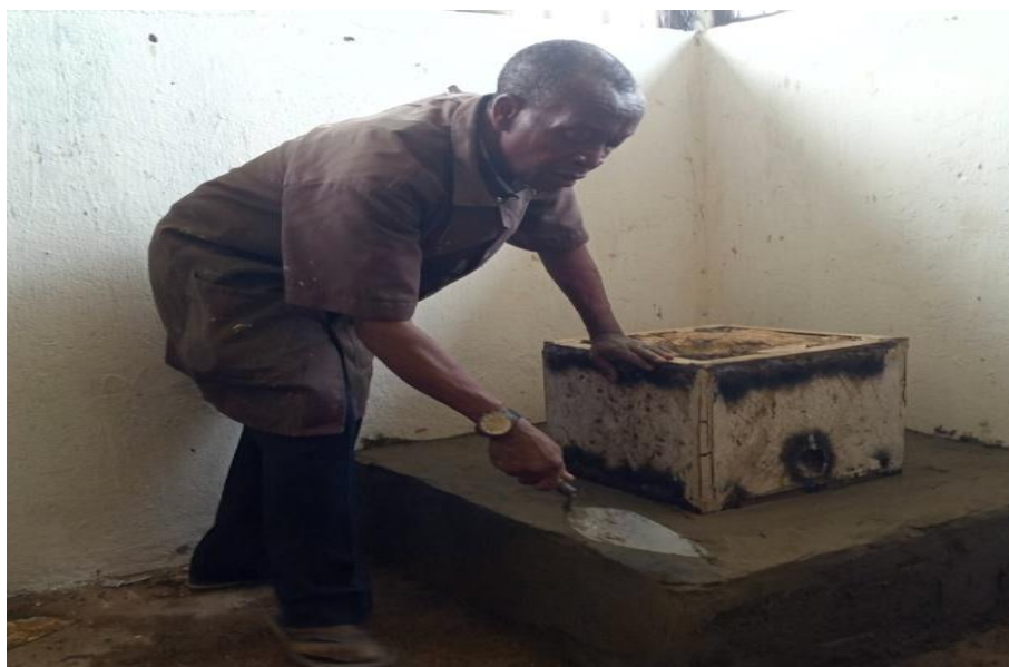
Figure 1: Stabilizing the Furnace
