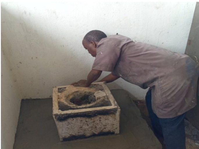
Figure 4: Furnace Base Preparation
