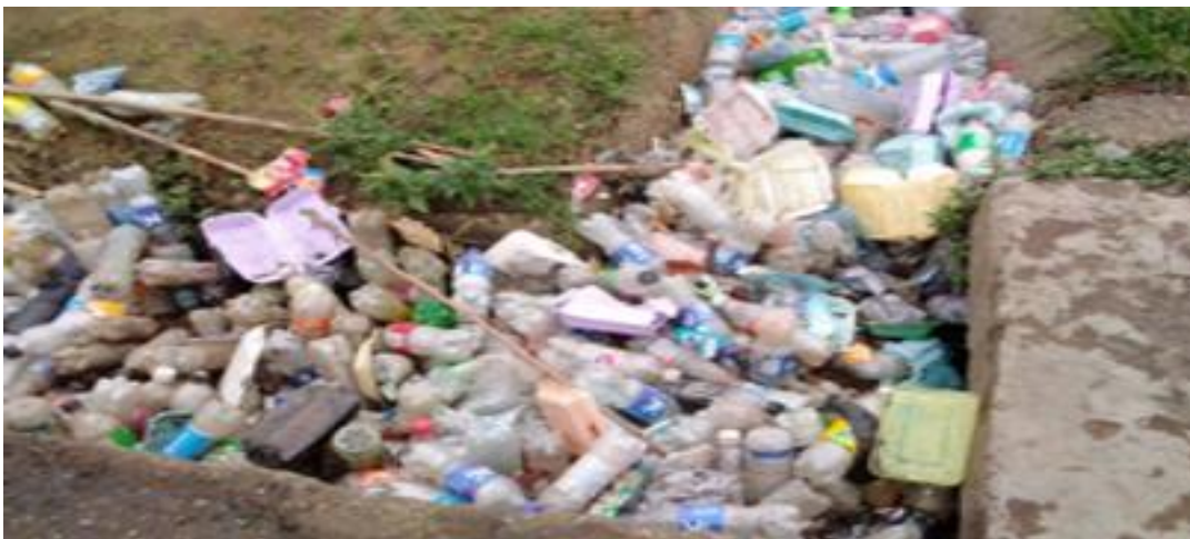
Figure 1: PET blocked drains
