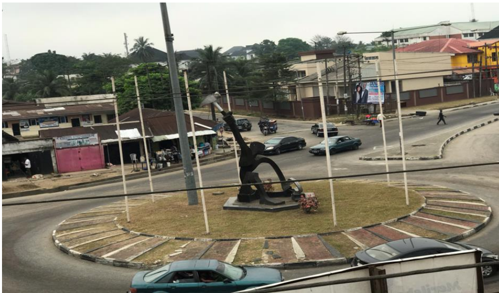
Figure 1: Area view of Effio-Ette Roundabout (ICD=18m)
