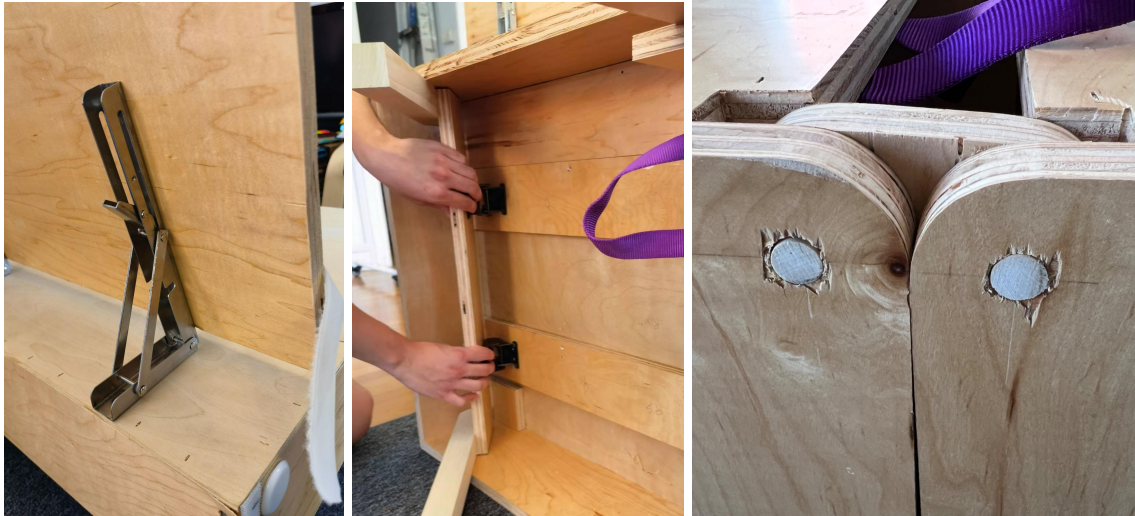
Figure 9: (a) Backrest joint , (b) Leg joint , & (c) Center linkage.
