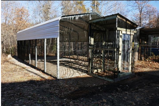
The finished enclosure.
