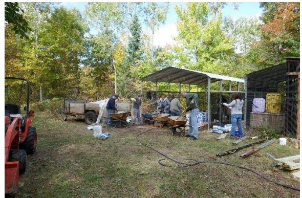
Mixing and pouring the concrete.
