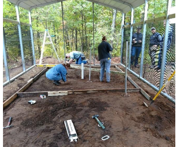
Digging the pond and making forms for concrete.
