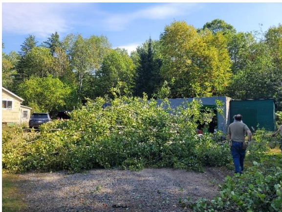
Clearing trees to ready garage for demolition.
