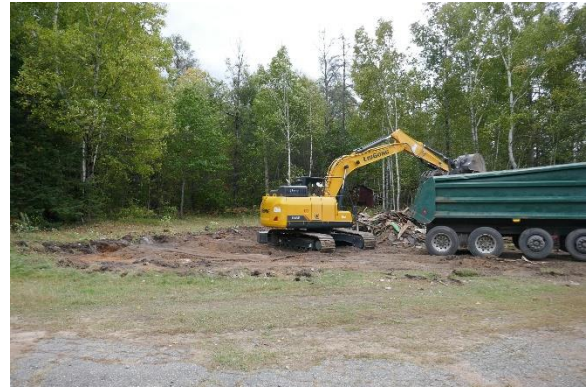
Garage gone. Ready for clean-up.
