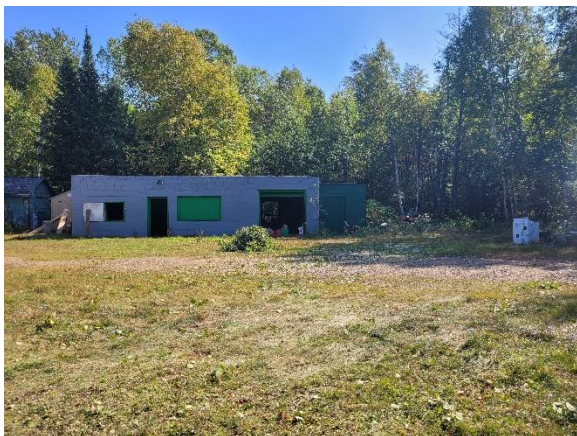
Garage ready for demolition.
