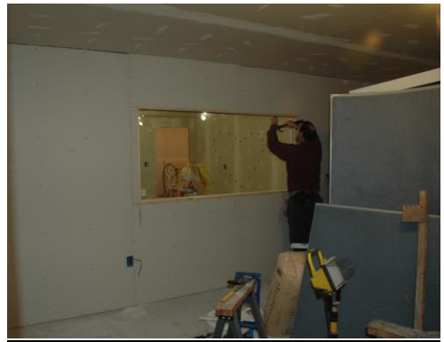
Viewing window into the nursery is installed
