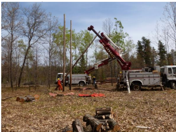
The first of poles go in the ground.
