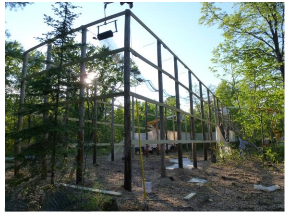
The framework is finished.
