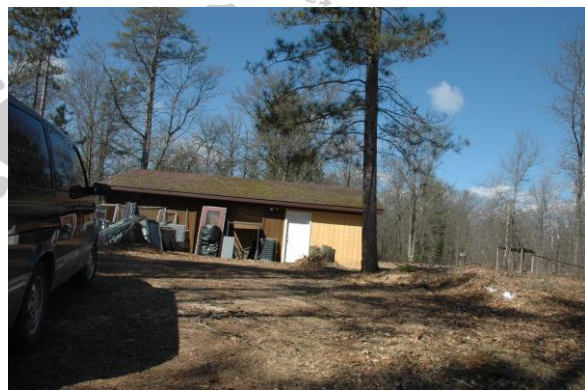
Garage with building site right and behind
