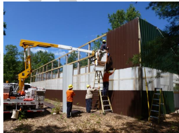
The last side of sheathing is going up.
