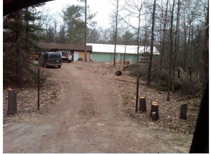
The shell of the main building is up. Photo taken 5/10/11
