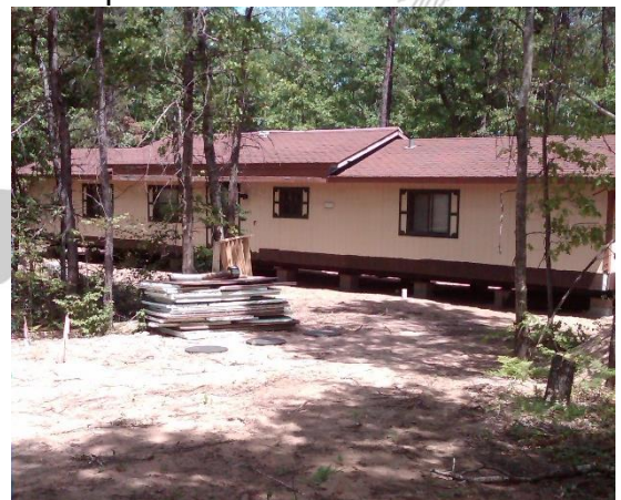
The mobile home for intern quarters/office is finally in place on site.
