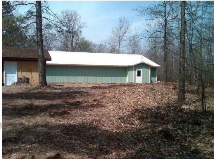
Monday, May 2 Drain Field Work Begins
