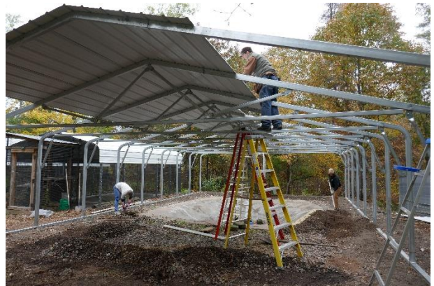
Roofing and gravel work.
