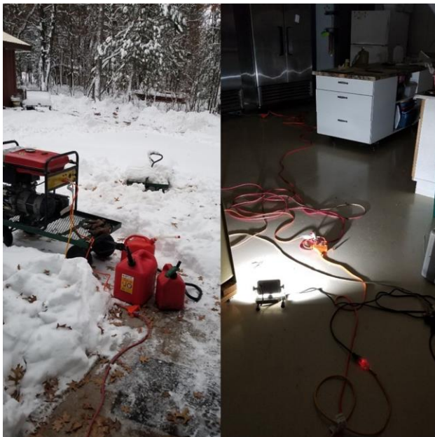
Generator outside the door, battery powered work light and extension cords were a way of life for four days.
