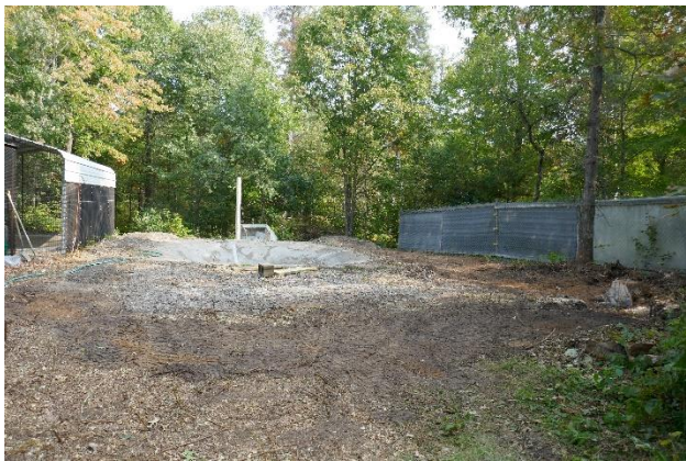
Old down, ready for the new to go up.
