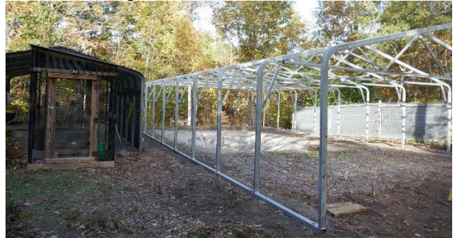
Side & roof framework complete.
