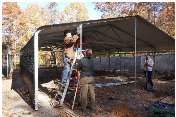
End walls being constructed.
