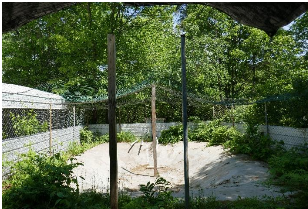
The roof readied for winter with supports to help with snow load.
