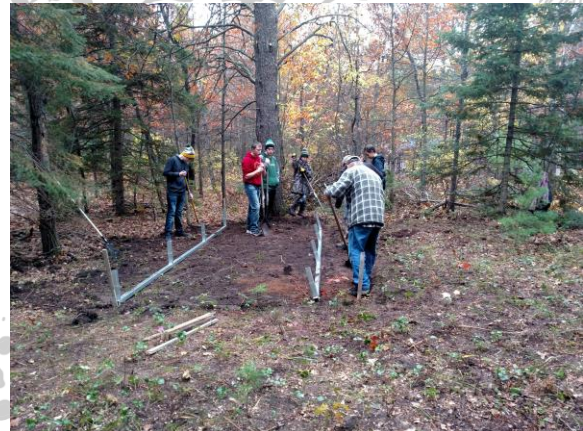
Prepping the site and setting up the base.
