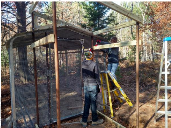
Working on the double door system.
