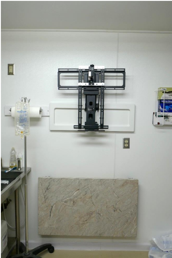
When not in use, the X-ray generator is stored away, and everything else folds out of the way against the wall.
