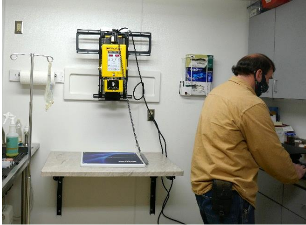
To use space the most efficiently, we modified a fireplace TV mount and built a drop-down table for our X-ray Suite.
