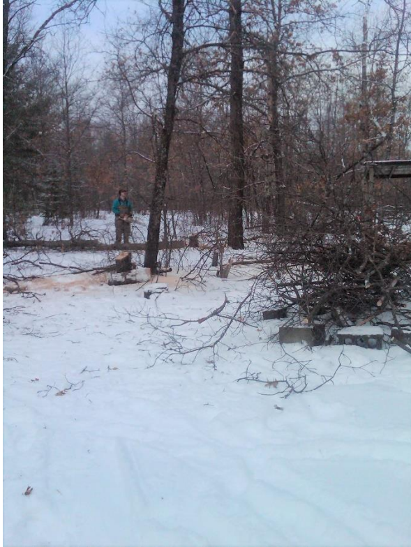
Clearing the building site. February 11, 2011.
