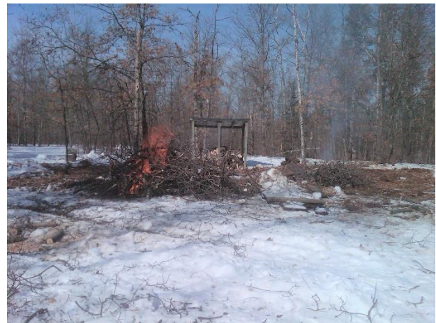
Burning brush cleared from building site. March 6, 2011.
