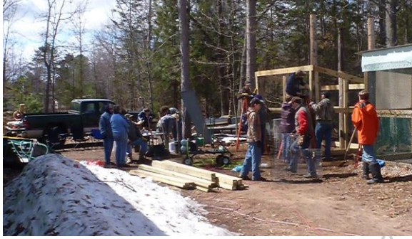
Frame going on the poles.
