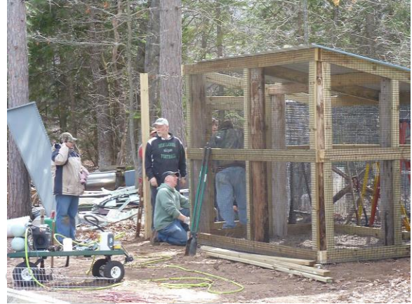
Working on the double door.
