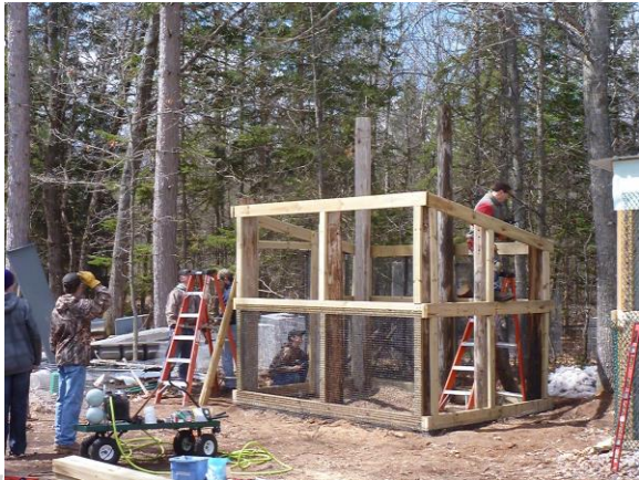
Preparing for the roof.
