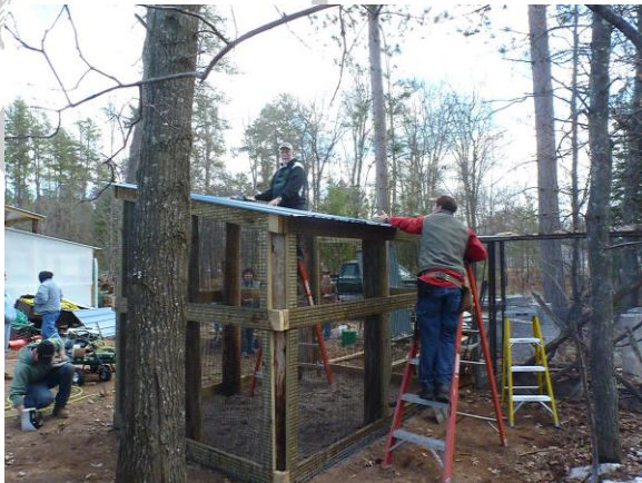
Installing the roof.
