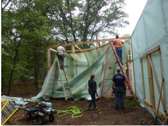
Installing fabric on the raptor complex.
