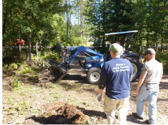
Stump removal to prepare for gravel.
