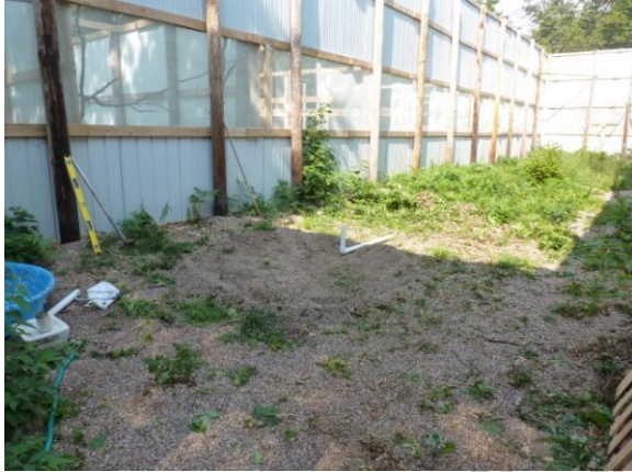
Roughing in the site of the new concrete pond.
