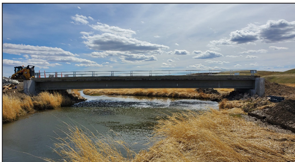
Figure 6: Ross Fork Creek Bridge, Judith Basin County. Constructed in 2021.
