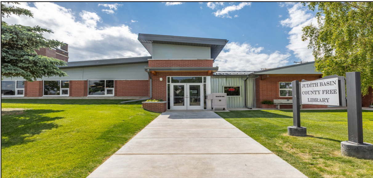
Figure 5: Judith Basin County Free Library (Diamond Construction, 2023)
