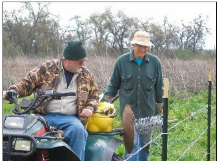
Hank Urbach and Warren Shaw stringing barbed wire during a China Creek fence building workday.
