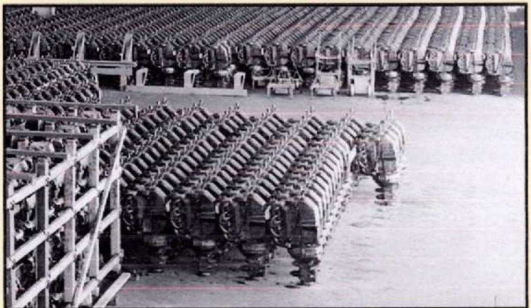
Era photo of Model A engines ready for installation at the Ford factory
