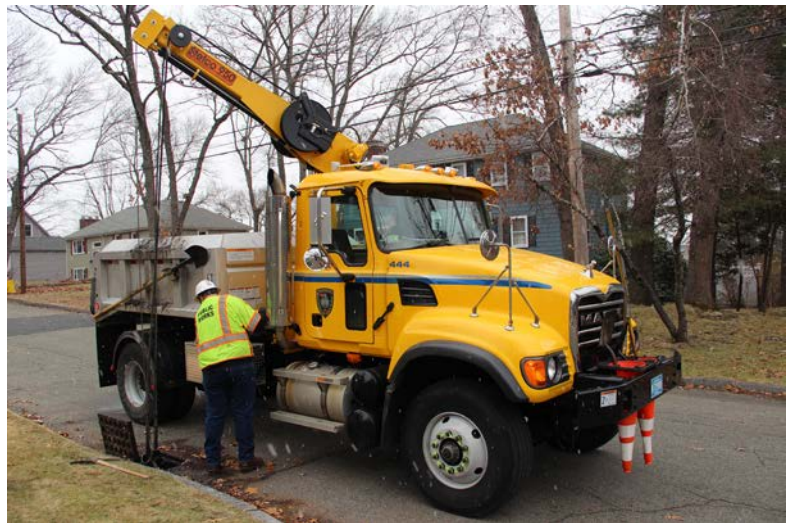
Cleaning one of the 10,000 catchbasins maintained by the Framingham DPW.
