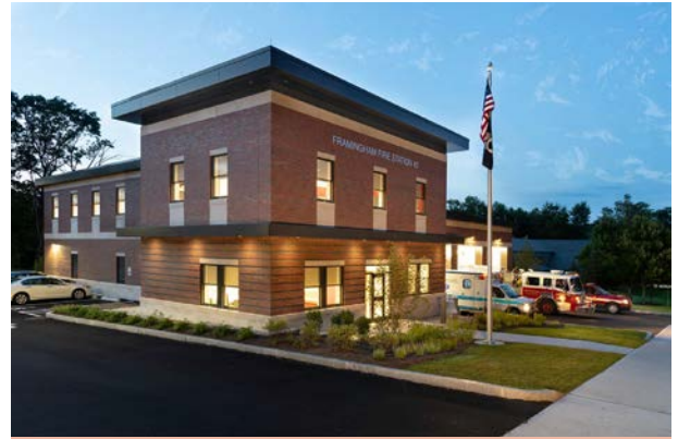
Framingham Fire Station #2
