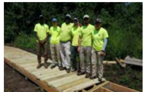
The 2019 Summer Conservation Crew constructing a boardwalk at 936 Central Street.
