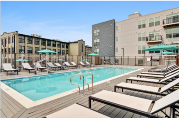
View of the new swimming pool at the Bancroft Lofts at 59 Fountain Street shows the renovated Bancroft Building in the background with the new construction in the foreground
