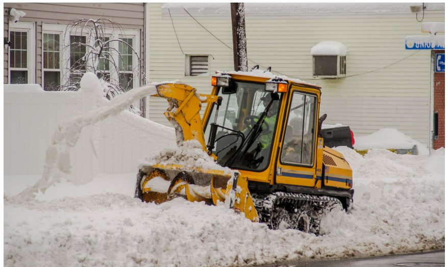
Clearing sidewalks on Union Avenue.
