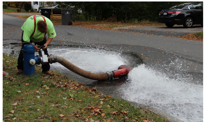
Hydrant Flushing, Fall 2020.
