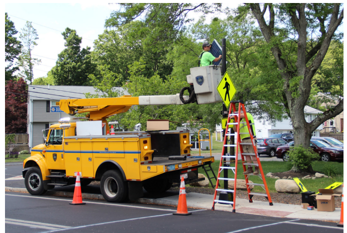
Rectangular Rapid Flashing Beacon (RRFB) sign installation on Summer Street.
