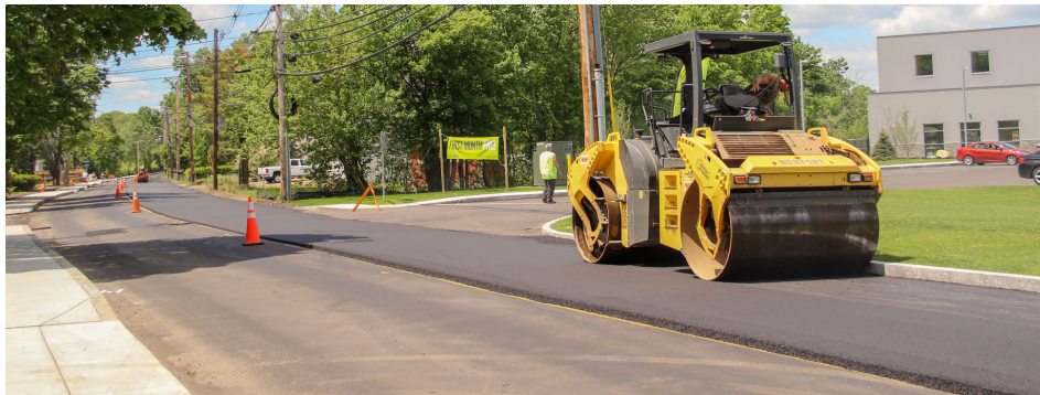
Leland Street Paving Operations.
