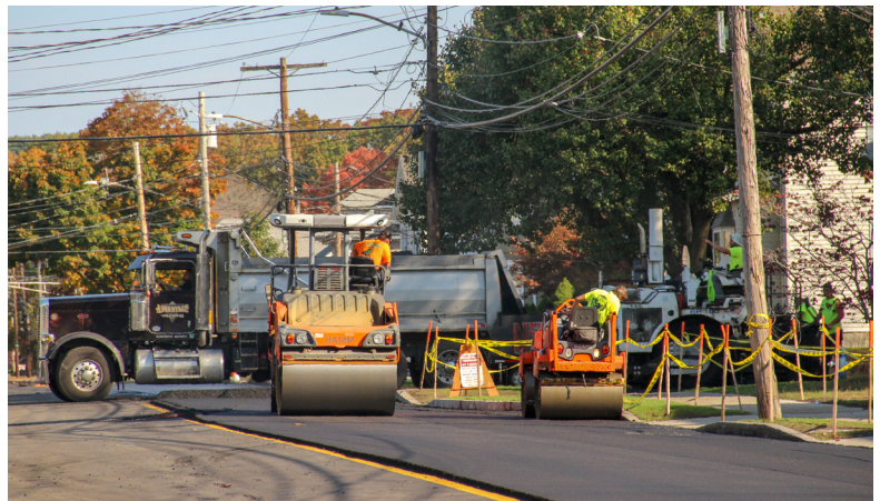
Grant Street Paving Operations.
