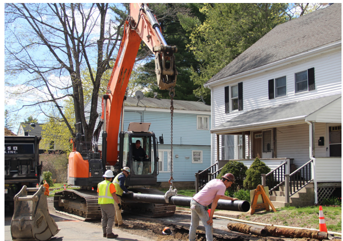
Replacing antiquated water main with new ductile iron pipe.
