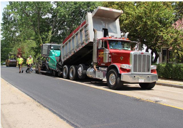
Surface Treatment on Dennison Avenue.
