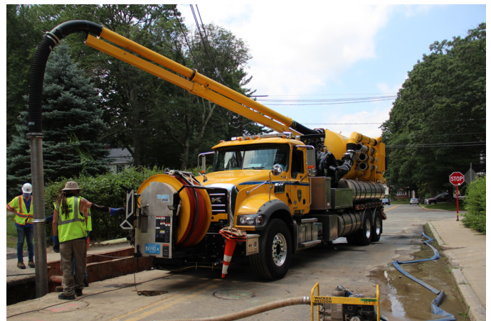
The Wastewater Department's vactor truck providing assistance.
