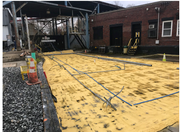
General Chemical Remediation Site
