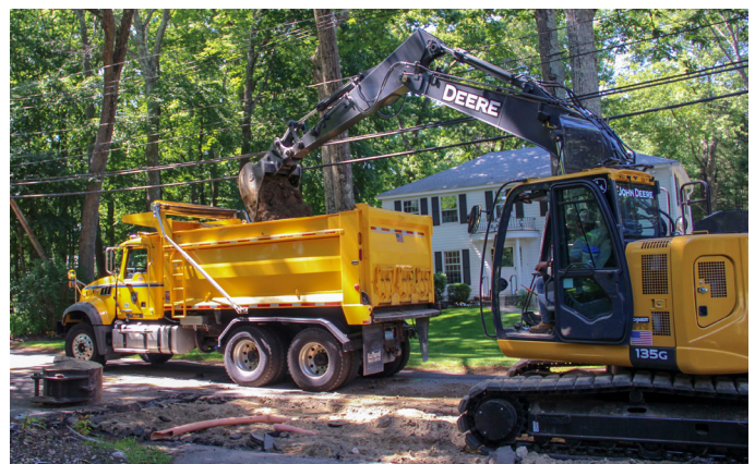
Excavating for sewer main replacement.
