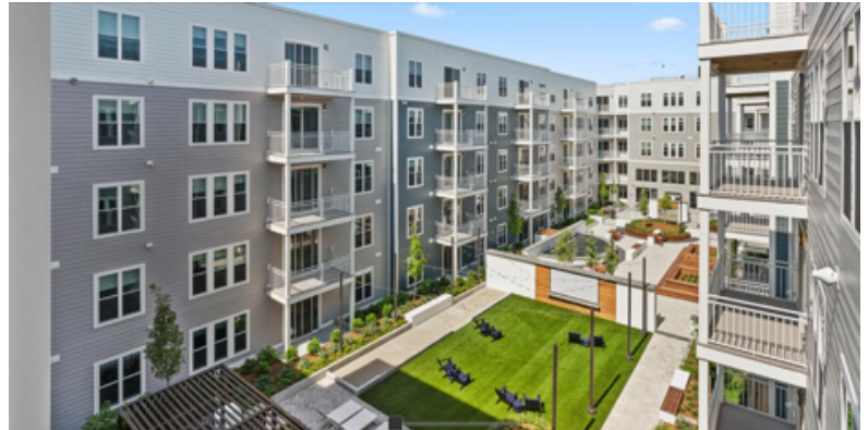
New courtyard amenity at the Modera Framingham at 266 Waverly Street
